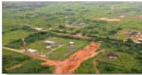
OML 4 F/S & Gas Plant
