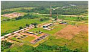
OML 41 Sapele F/S & Gas Plant
